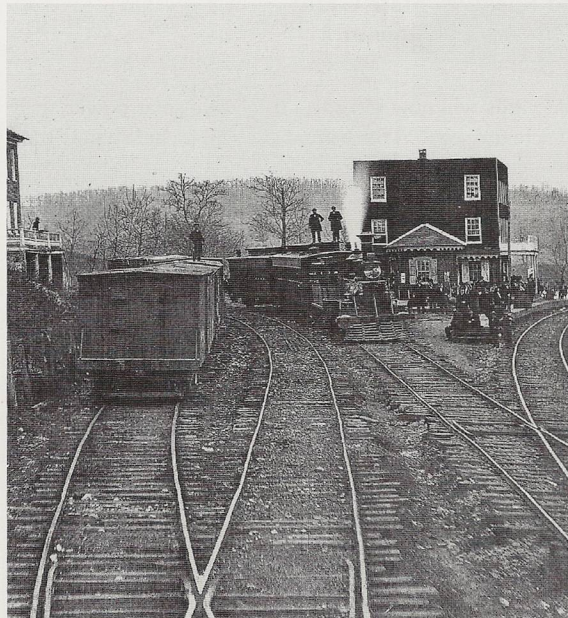
Hanover Junction, Pa., November 1863. The NCR track is to the right of the station and the Hanover Branch RR to the left. (Matthew Brady photo)
